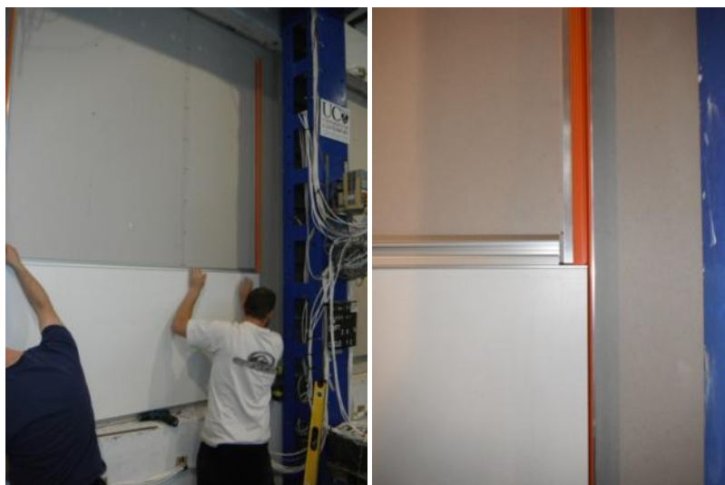
Figure 4.4. WEDGE 02 Specimen. Plastic vertical jointing elements located in the vertical gaps.
